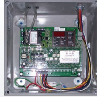
Dust collector pulse system
