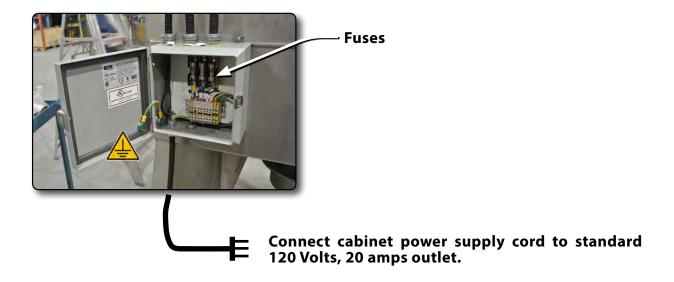
All electrical connections to the ISTblast cabinet should be made by a qualified electrician and must complied to the codes, standards, and procedures specified by the local authority having jurisdiction.
