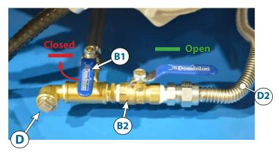
Close the ball valve [B1], open the ball valve [B2] unscrew the plug [D], connect it to a pump and drain the oil from the boiler
