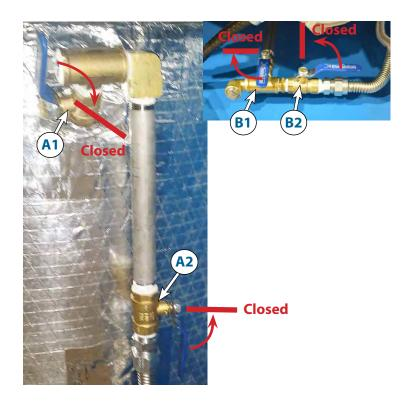
Close the 4 ball valves at the boiler level top [A1] [A2] and at the bottom [B1] [B2]
