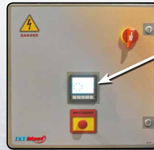
HMI* touchscreen control
