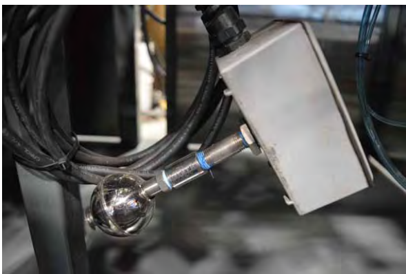
Fig. 2 - Sludge Discharge Float Switches
