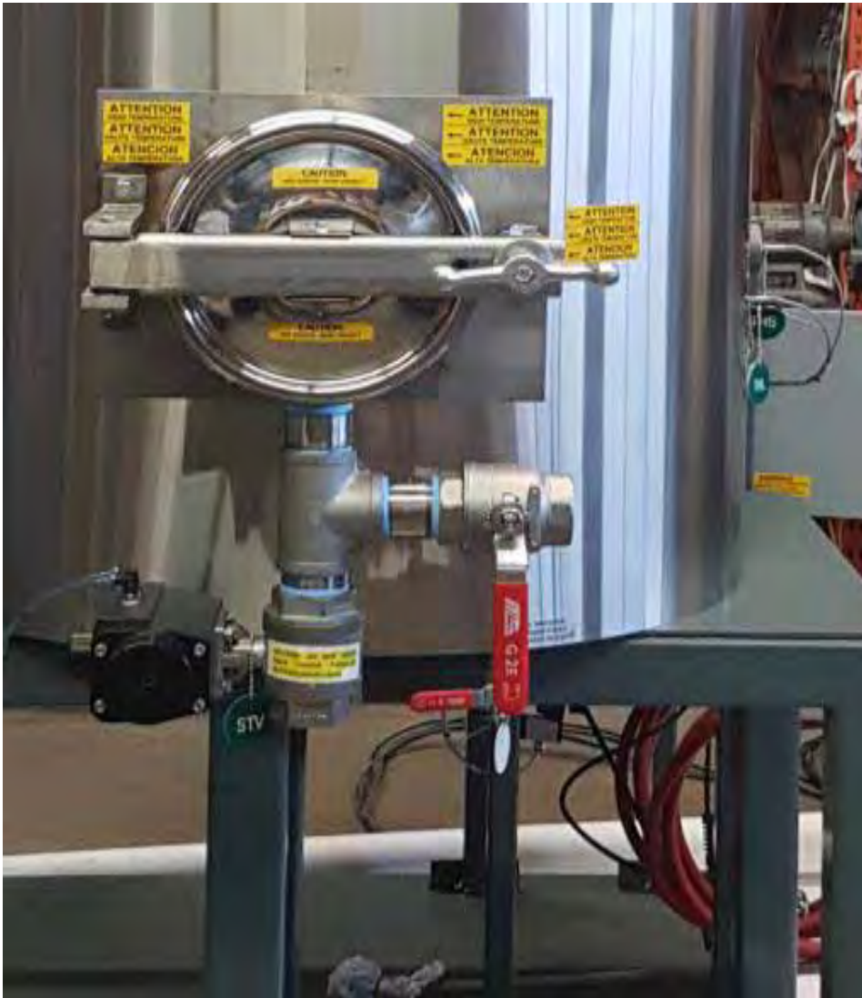
Fig. 5 – Pneumatic Drain Valve (STV)
