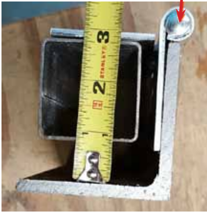
When the joint expands, it will have a thickness of 7/8". Allow time for the joint to expand.
