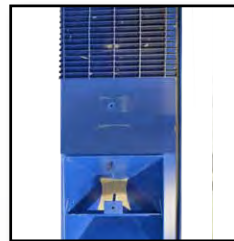
Pneumatic recovery system with floor hoppers
