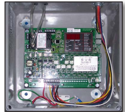
Automatic Pulse Cartridge Cleaner. A light illuminates to indicate when the cartridges must be replaced.
