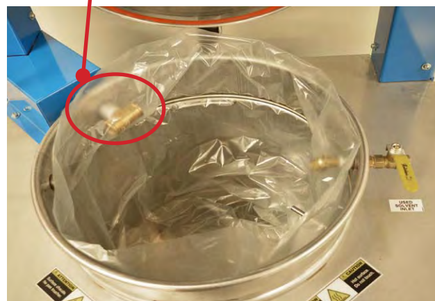
Wrong installation (Bag above the elbow)
